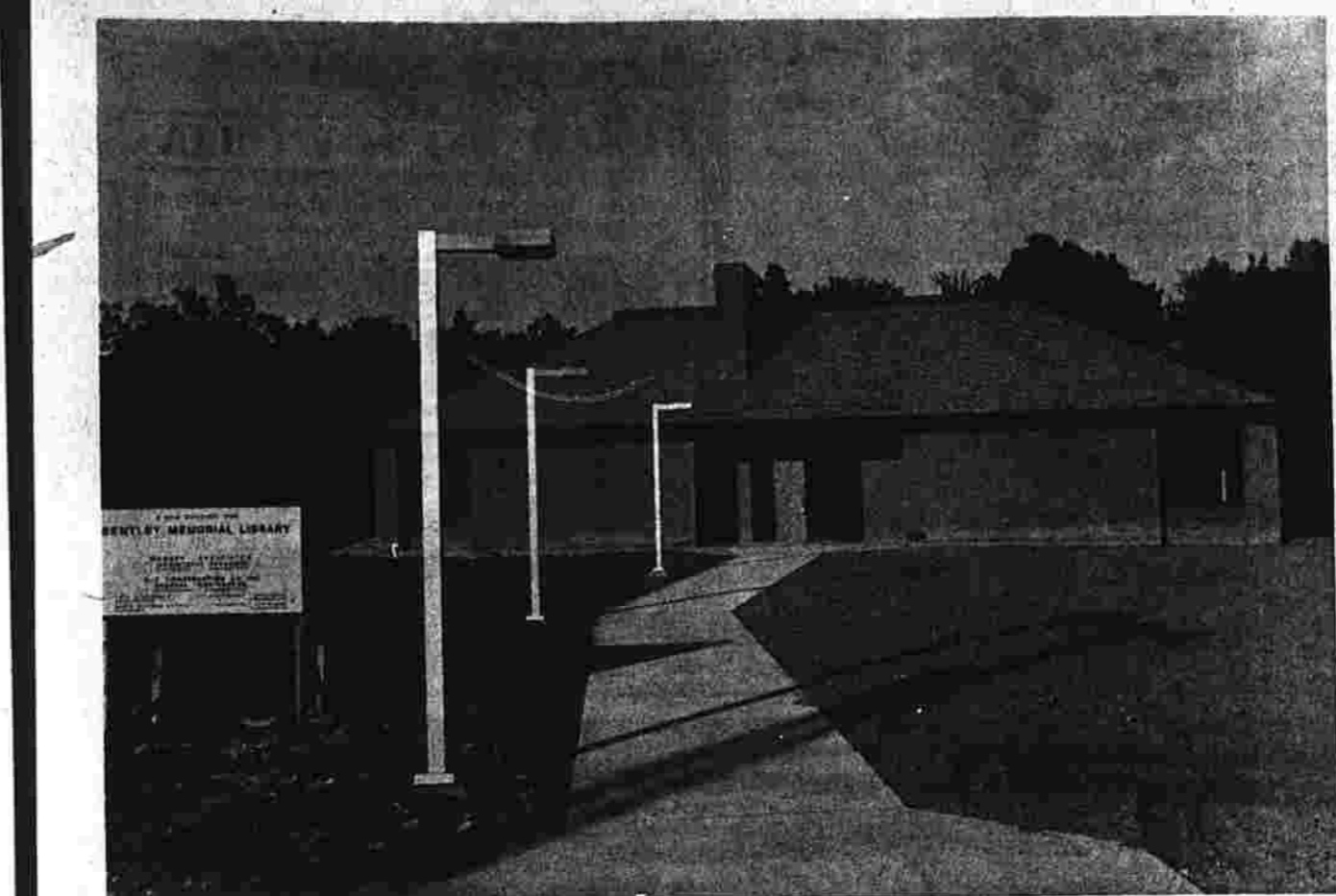
Bolton's new public library nearly complete
